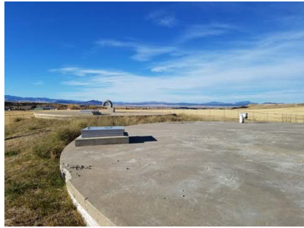
McClellan Storage Tanks
