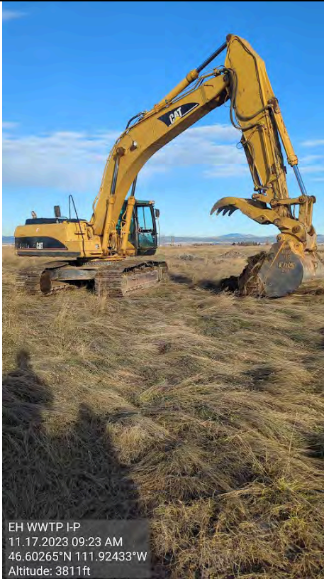
Picture # 1: CAT 330C Excavator
