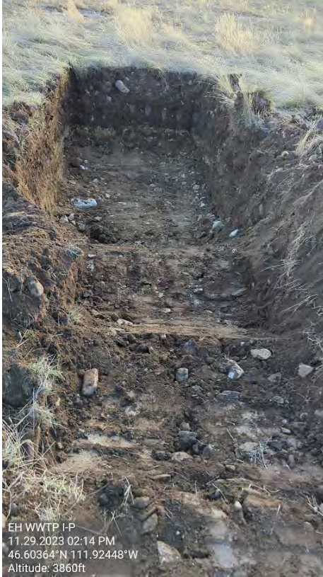
Picture # 9: Infiltration test location
