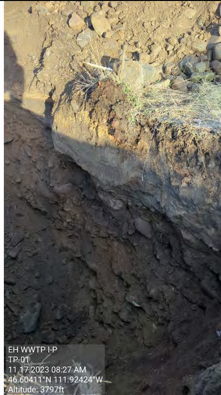
Picture # 2: TP-01 Overview
