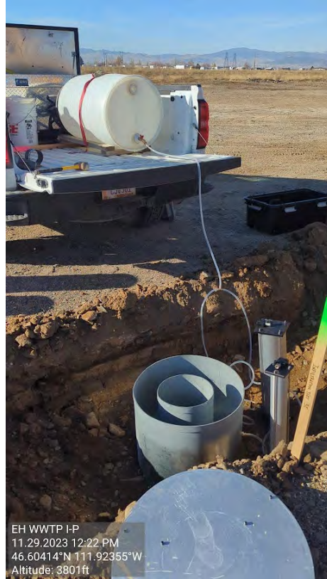
Picture # 10: Infiltration test setup
